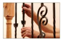
23. Firmly tighten the set screw on the bottom socket to secure the baluster. With both hands turn the baluster counterclockwise to back it securely into the handrail hole.
