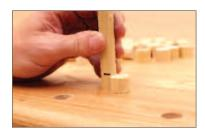
5. The 3/4" holes need to be plugged with the included dowels. Measure the depth of the hole to ensure the dowel will fit up to 1/16" below the tread surface. Example: Insert a rod into the hole and mark off above the recommended depth (See # 9 for installation).
