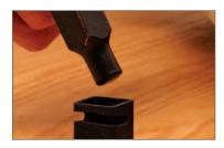
Now measure the baluster for cutting. It is important to invert the baluster and place it into the socket.
