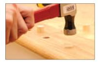
Tap the dowel into the 3/4" hole and make sure the dowel sits flush with the tread or no more than 1/16" below the surface.
