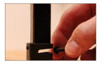
17. With the baluster raised into the handrail hole, insert the baluster support axle into the socket. Firmly tighten the socket set screw. Then, with both hands turn the baluster counterclockwise to back it securely into the handrail hole (See # 23).
