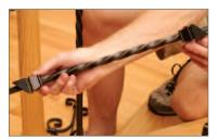
15. Before installing the 30" knee wall baluster, position the Top Angle Shoe and Base Angle Shoe on the baluster so that they each match the angle of the handrail and baseplate.
