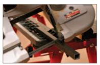
15. Cut the baluster at the point shown in # 14. We recommend renting a portable band saw for the cutting process. TIP: Always cut balusters slightly longer and adjust the cut shorter to avoid wasting a baluster.
