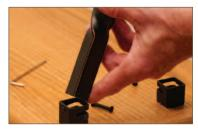
17. Insert the baluster into the socket.
