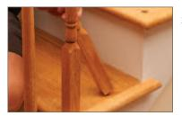
Remove the old balusters from the previous installation to reveal the installation holes in the tread and the underside of the handrail.
