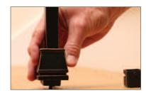
22. Now that the baluster has been raised, drop the Base Flat Shoe to the tread surface.
