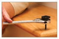
11. Use a crescent wrench\* (as shown) to screw sockets into each dowel hole on the treads. The sockets must sit flush with the tread.
