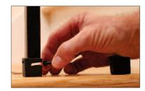
With the baluster raised into the handrail hole, insert the baluster support axle into the socket.
