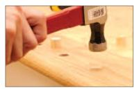
Tap the dowel into the 3/4" hole and make sure the dowel sits flush with the tread or no more than 1/16" below the surface.
