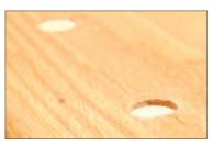
This picture shows how the dowel plug should be correctly installed—flush with the surface or no more than 1/16" below. Let the epoxy glue set and cure.
