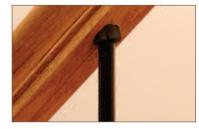
24. At this point ensure that the top of the baluster has pushed the bushing up into, or as far as possible into the handrail hole (See # 21). This will firmly secure the baluster in place.
