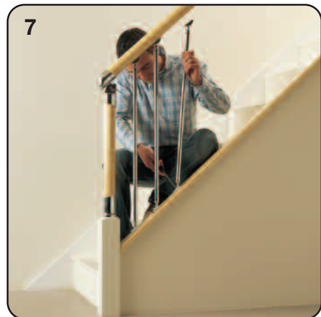
7 Begin fitting the balusters.
