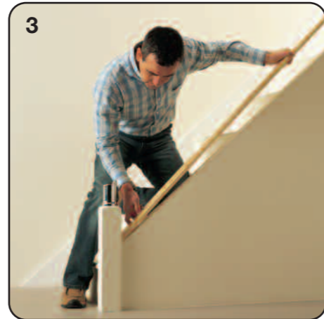
3 Measure and fit the baserail (this process differs for closed or open string staircases, see full fitting instructions in newel base connector for details).
