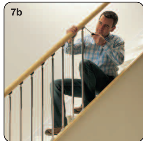
6 Fit the handrail to the correct angle using the top connector on the top post.
