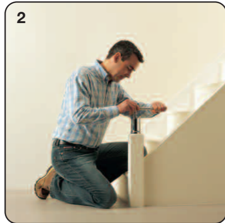
2 Secure the newel base connector onto the newel base using the fixings provided. Repeat steps 1 and 2 for all newel bases.
