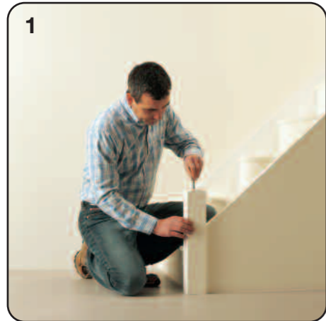
1 After drilling your newel base, attach the threaded bar through the base into the barrel nut.
