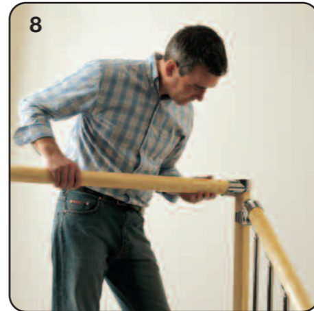
8 Begin fitting appropriate landing balustrading.
