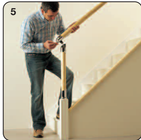
5 Attach the handrail using the bottom connector.
