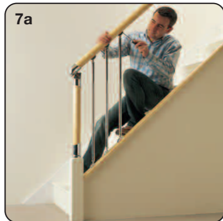
7 Begin fitting the balusters.
