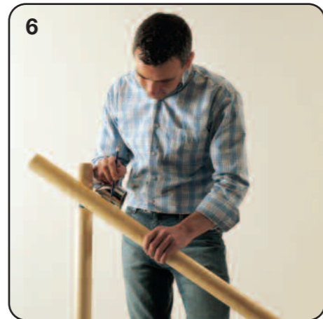
6 Fit the handrail to the correct angle using the top connector on the top post.
